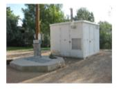
The Bus Barn electric service includes single phase power converted to 3-phase. The back-up generator is also single phase, requiring a phase converter to operate this station from the grid or generator. This project includes running 3-phase power to the facility and modifying the generator to 3-phase (or generator replacement if necessary). The Taft Lift Station needs new rails, wetwell coating, and new hatch/lid.
