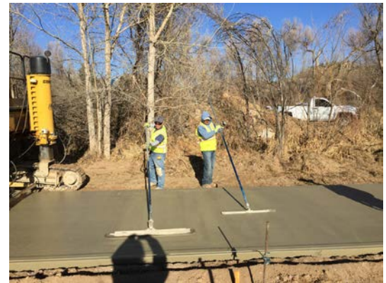
Trail construction at Rossum Drive connection
