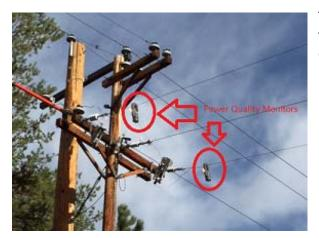
The devices circled in the picture to the left are used to monitor the quality of power that is delivered by the City of Loveland to the customer or end user. These devices are highly accurate in monitoring voltage, current, KWH, and power factor.
