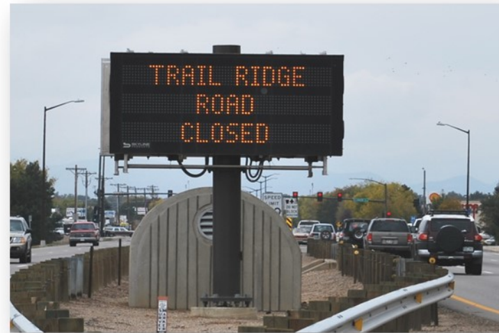
VMS – BUTTERFLY STRUCTURE – US 34/DENVER AVE. – Back to back signs for east/west traffic
