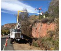
Several poles along the north side of Highway 34 are in areas that have limited and restrictive access and have proven difficult for crews to work on. Power Contracting was able to track down a bucket truck with a 75' plus boom that allowed them to work on the old and new poles from the shoulder of Highway 34. This expedited
