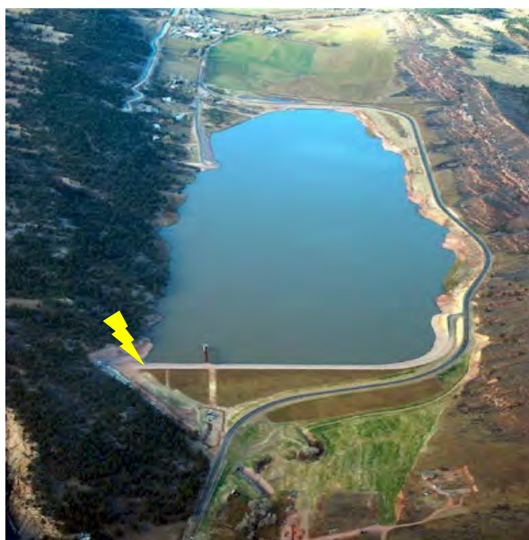
Figure 12 Proposed installation location for the Eco2 Speece Cone at the Green Ridge Glade Reservoir
