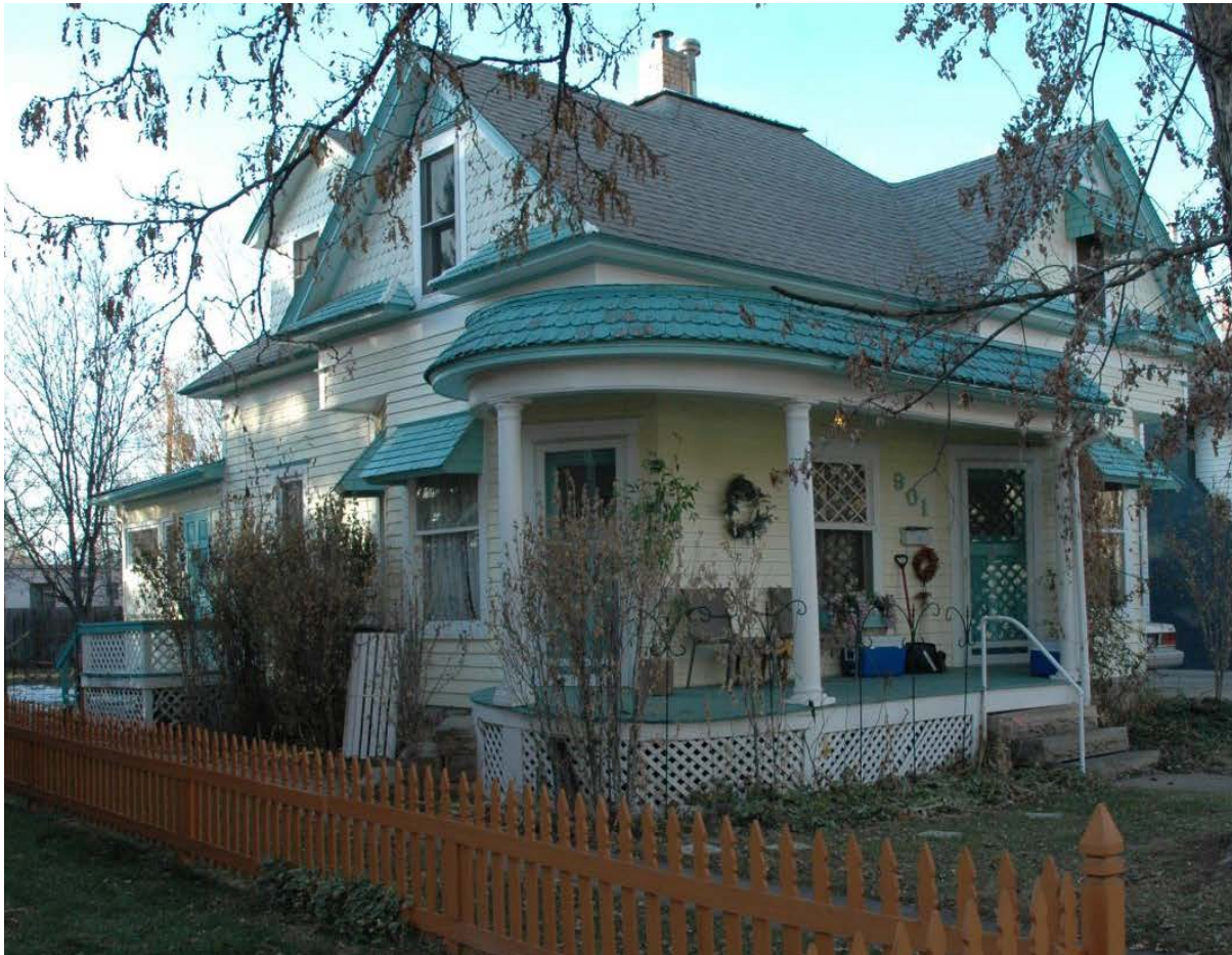
South and East Elevations
