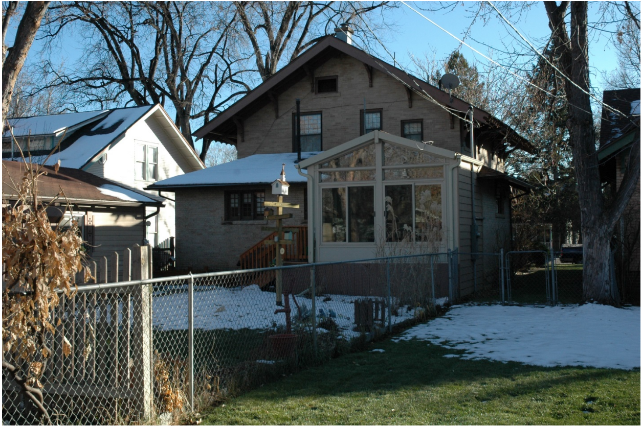
Figure 4: North (Rear) Elevation
