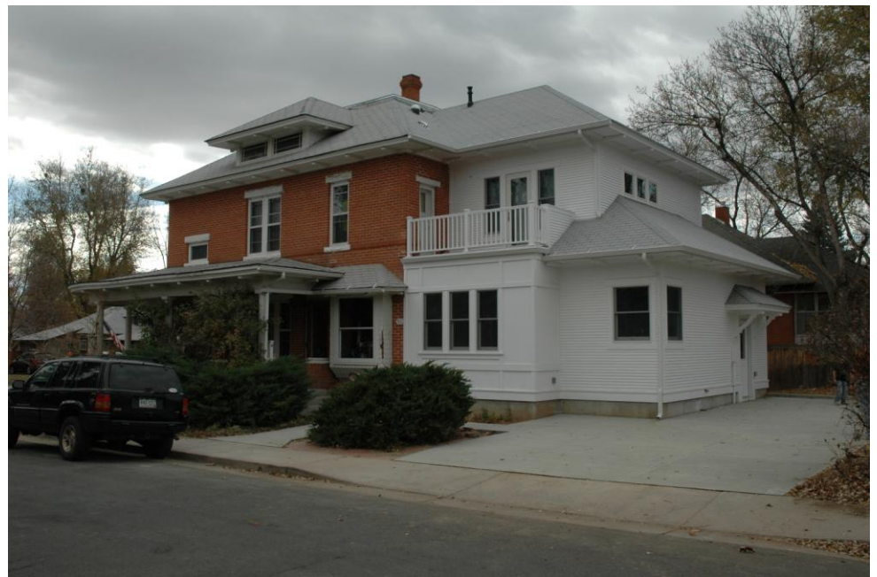
From Northeast (showing addition)
