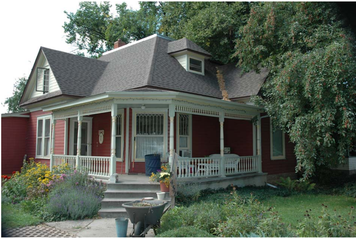
Picture 1. North elevation.
