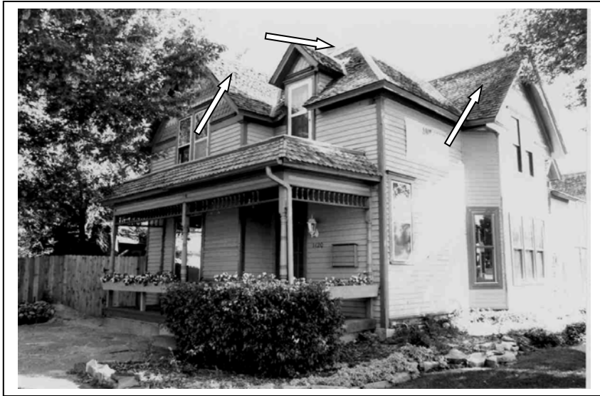
Photo #4. Features include intersecting gables, truncated hip roof.
