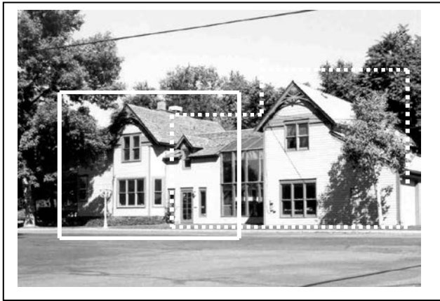
Photo #7. Dashed line shows 1983 addition. Solid line shows area of original DeGroat/Sisk House.
