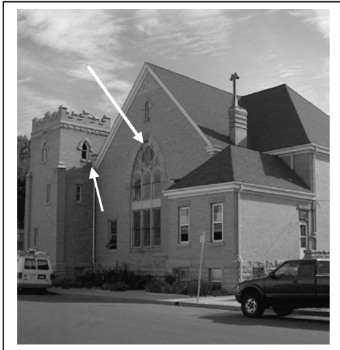
Photo #5. Gothic windows on west elevation. Tracery is found in the upper portion of the large window.
