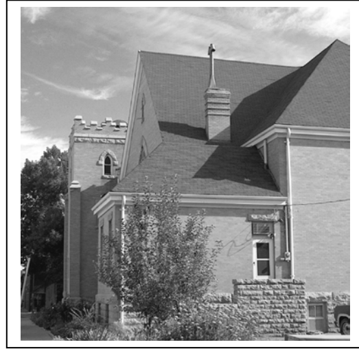
Photo #6. Broad-planed, steeply pitched roof and mottled pressed-brick is characteristic of Gothic Revival style.
