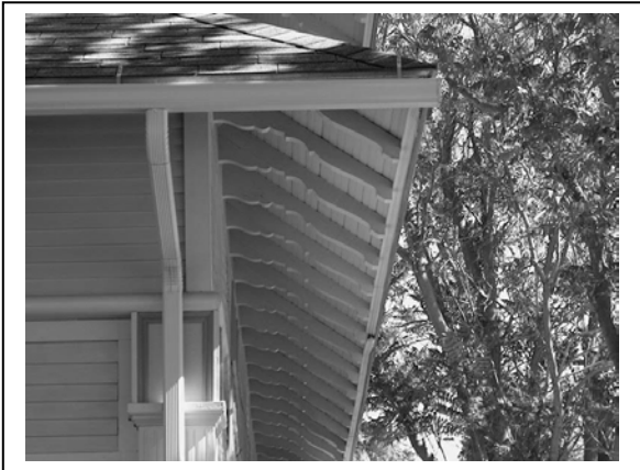
Photo #5. Sculptured wood rafters beneath wide overhanging eaves.
