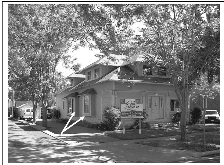
Photo #7. West elevation with boxed bay windows.
