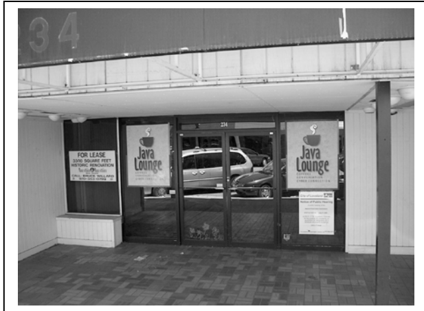
Photo #5. Current configuration of storefront with deeply recessed entry bay and tiled floor.
