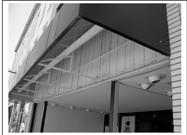
Photo #6. Clerestory covered with wood paneling and awning.
