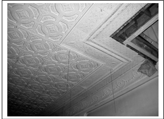
Photo #10. Pressed-tin ceiling panel detail.
