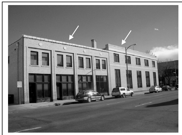
Photo #4. West elevation shows front-block, and lower height rear-block.
