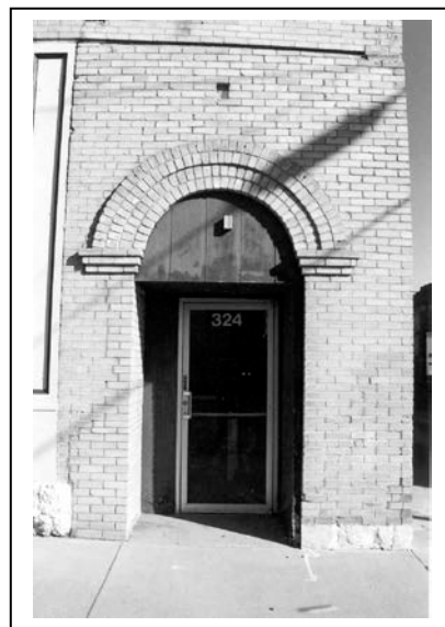
Photo #11. Recessed, arched entrance located on west elevation, Cleveland Avenue, with arcaded brick corbels.
