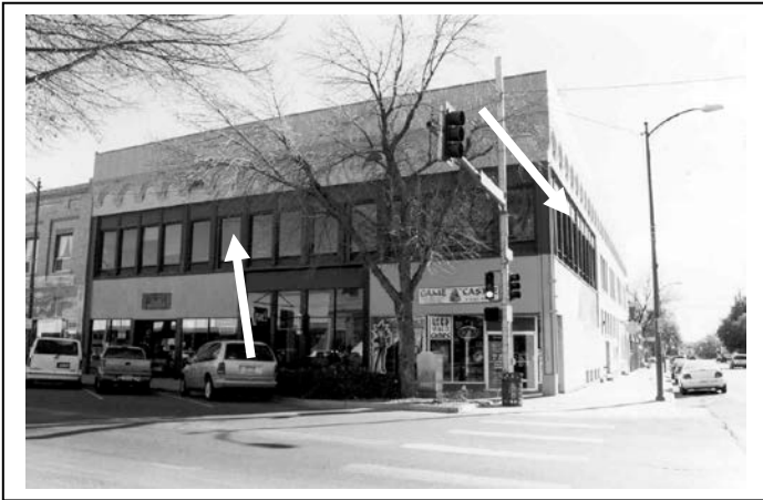
Photo #8. Second story windows with sealed transom and bottom panels resulting from 1970's renovation. (photo taken 2003).
