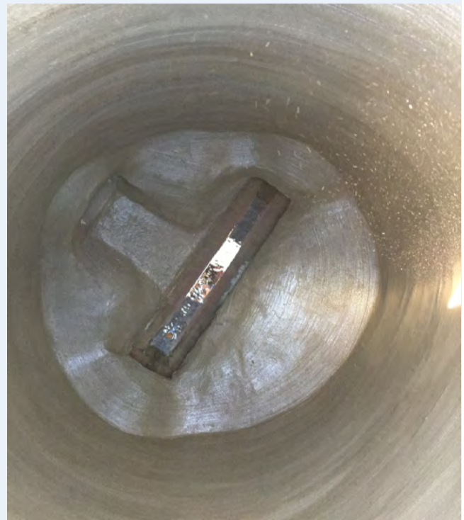
The rehabilitated manhole will now better withstand the elements due to a new coating which seals the old brick.
