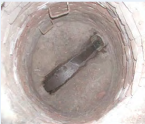
This old manhole , constructed of bricks and mortar, was in serious need of repair.
