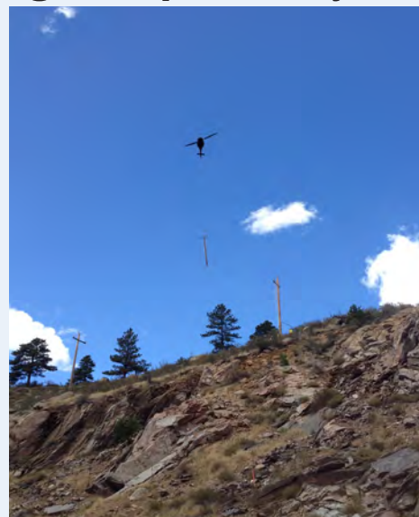
A helicopter lowers a 700-pound pole on the ridge near Viestenz-Smith Mountain Park. This process will be repeated many times over.
