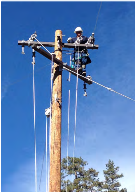
Lineman Justin Buxbaum holds steady on a crossarm approximately 40 feet off the ground as he strings and guides electrical wire from pole to pole along the ridge of the canyon.
