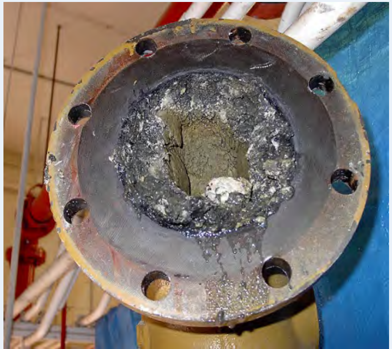
The result of fats, oil and grease (F.O.G.) are seen in this Loveland sewer line.
