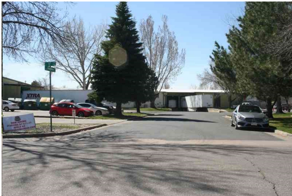
View of typical light industrial development along Josephine Court located south of the subject property.
