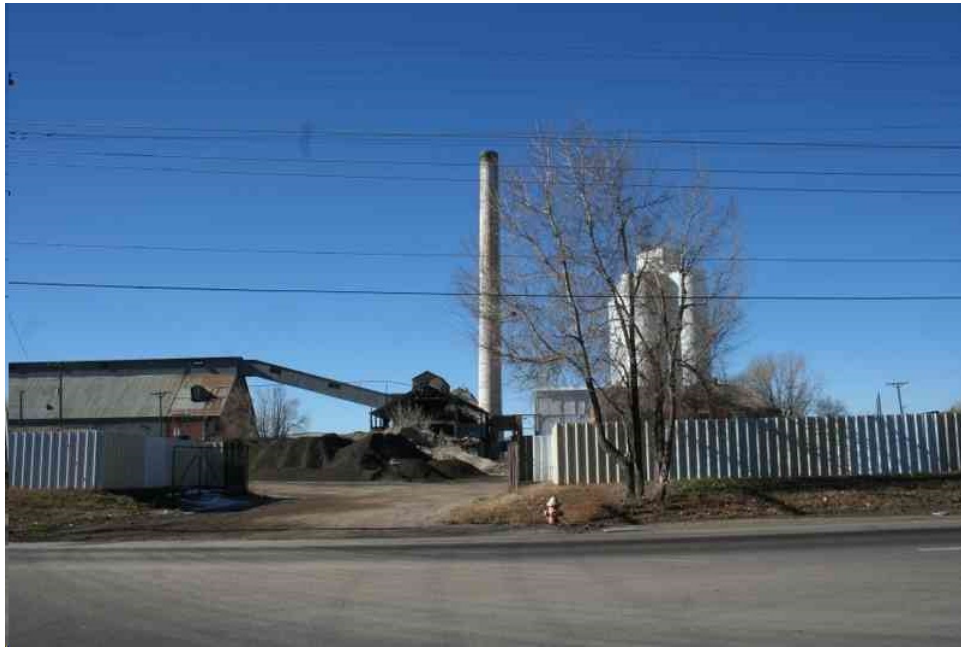
View of the former Great Western Sugar Factory located west of the subject property.
