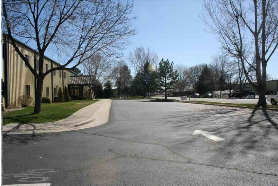
View of the parking and access area located on the front (south side) of the building.
