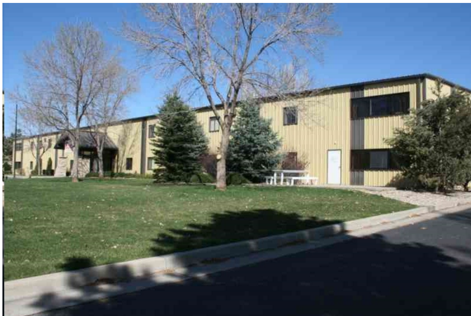
Front view of the subject property looking northwest from East 11 th Street.
