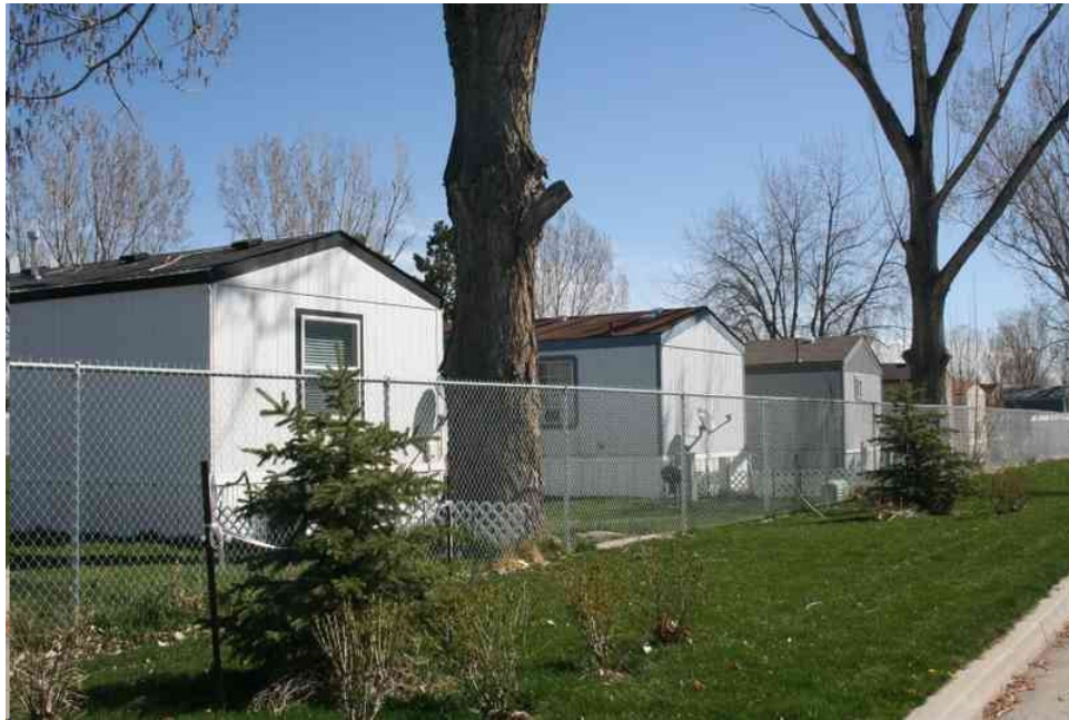
View of a mobile home park located north of the subject property.
