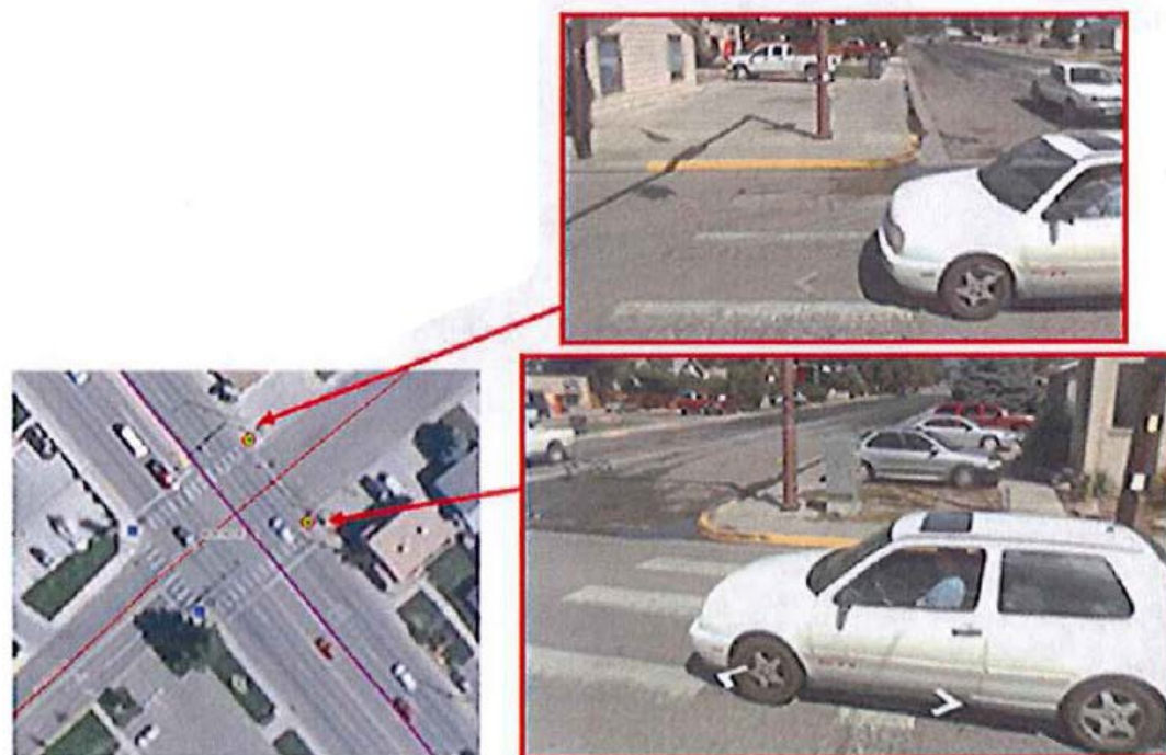
Figure 3 - Sidewalk and crosswalk without curb ramp
