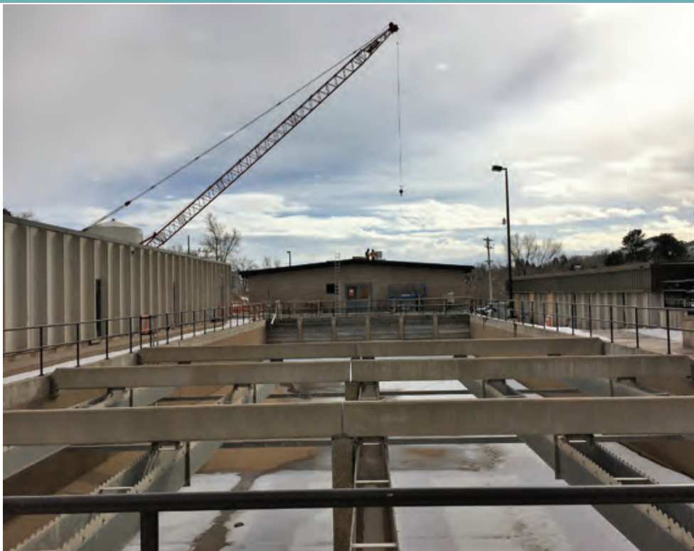
A view looking south across the sediment tanks dating from 1940, above, shows the new 8 MGD filter plant. Below, a 22,000 gallon tank in the new west chemical building was taking shape.
