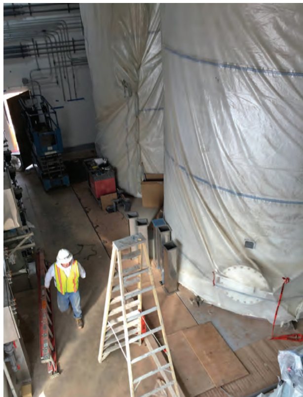
A view looking south across the sediment tanks dating from 1940, above, shows the new 8 MGD filter plant. Below, a 22,000 gallon tank in the new west chemical building was taking shape.
