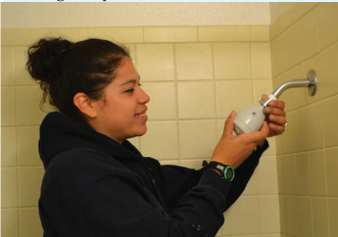
Another corpsmember installs a ‘low-flow,’ water-saving showerhead in a homeowner’s bathroom.
