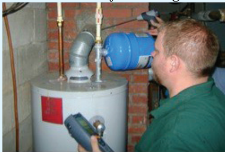
A home energy auditor tests a water heater to make sure it's operating properly.
