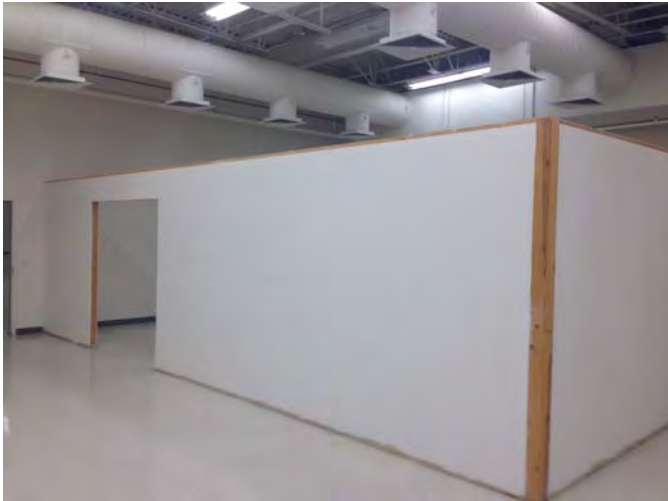
Co-location area- partitioned office area.
