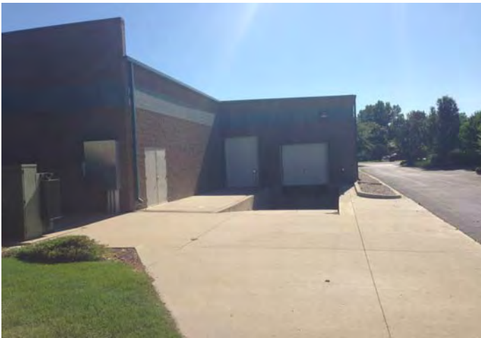
Drive-through and dock-high doors located on the southwest corner of the building.
