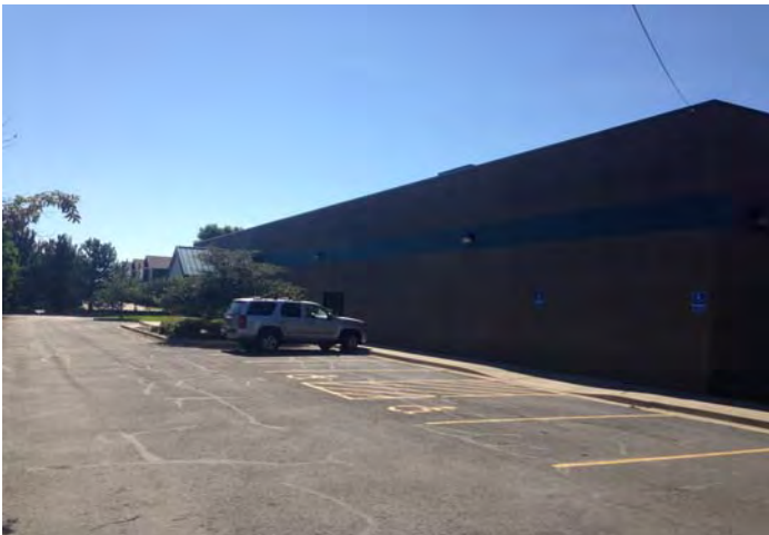
North elevation looking southeast.
