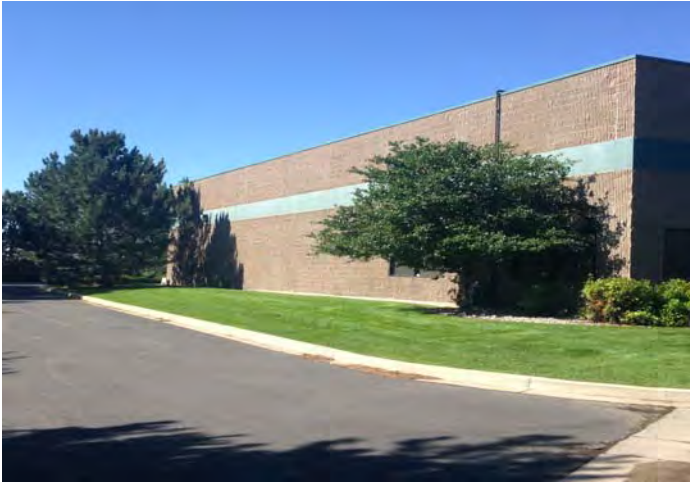
West elevation looking northeast.
