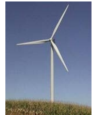
Structural health monitoring
