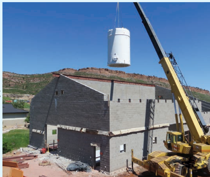
The new West Chemical building at the treatment plant will house a 22,500 gallon tank that holds the solution used water disinfection.
