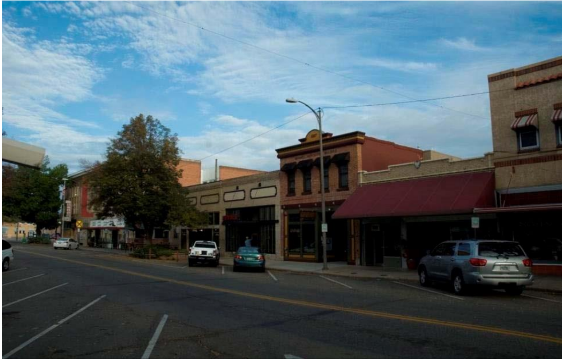
Photo 11: Camera facing northwest -103/111/117 East 4th Street, 119 East 4th Street, 121 East 4th Street, 125 East 4th Street, 129 East 4th Street, 133/135 East 4th Street – 5LR.685 C, 5LR.5076 NC, 5LR.6176 C, 5LR.5077 C, 5LR.6175 NC, 5LR.5075 C
