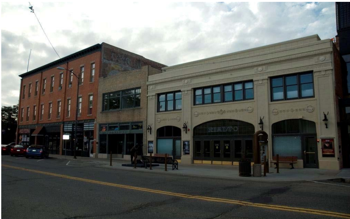
Photo 18: Camera facing southeast - 228 East 4th Street, 234 East 4th Street, 236/238/248 East 4th Street - 5LR.1058, C, 5LR.5069 C, 5LR.1059 C
