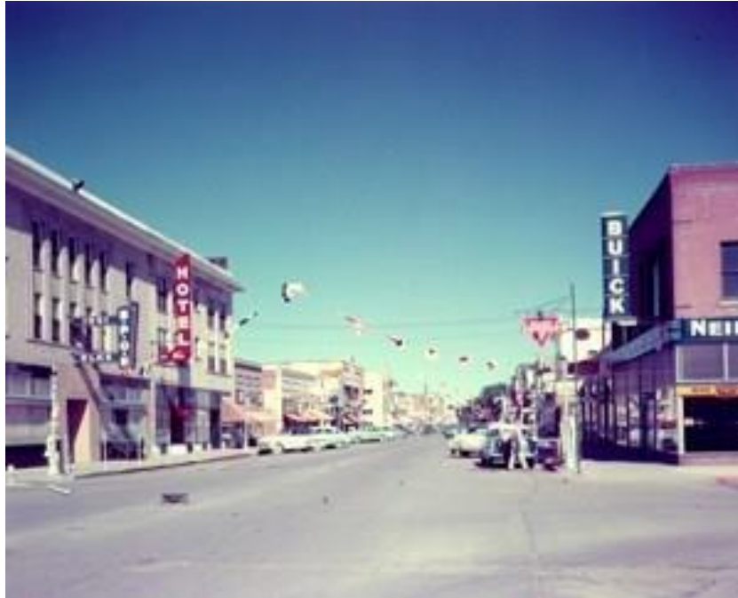
Figure 10: 100 block of 4th Street, view to E. ca. 1955. Courtesy Loveland Public Library, Loveland, Colorado.
