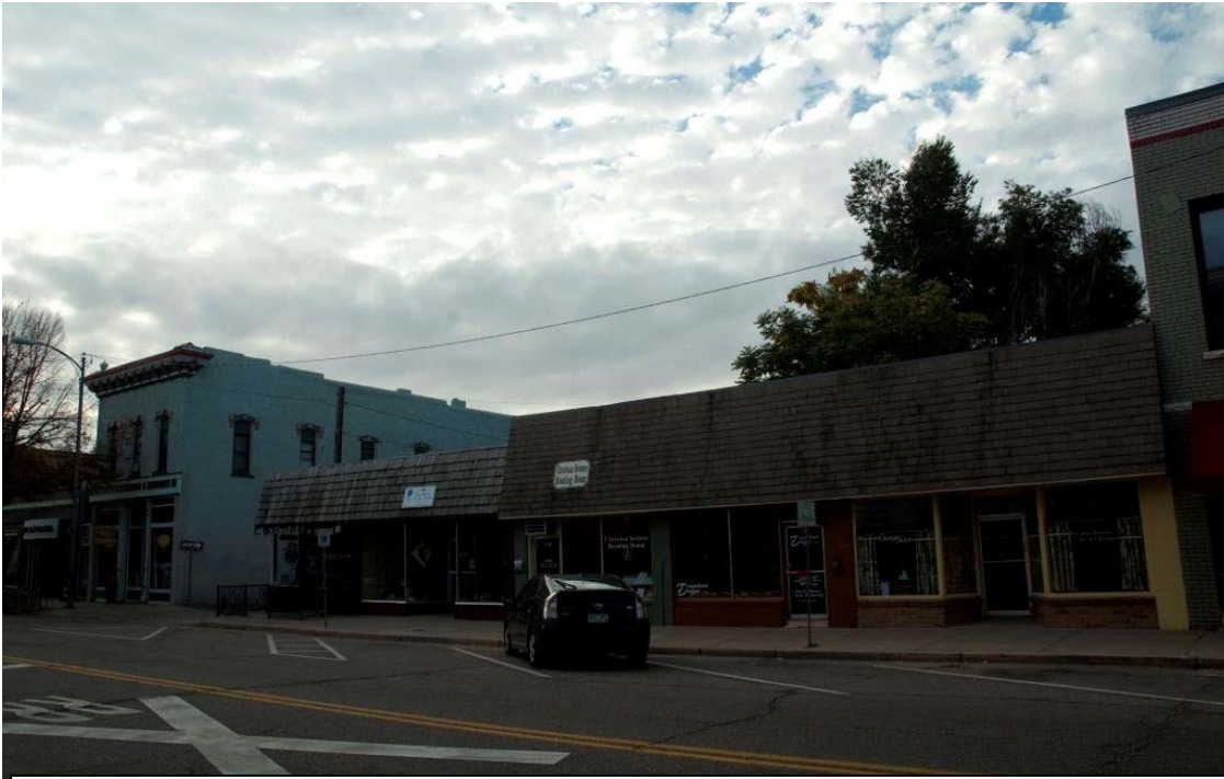
Photo 15: Camera facing southeast - 110/112/114 East 4th Street, 116/118 East 4th Street 120/122 East 4th Street - 5LR.6178 C, 5LR.6179 C, 5LR.5065 C
