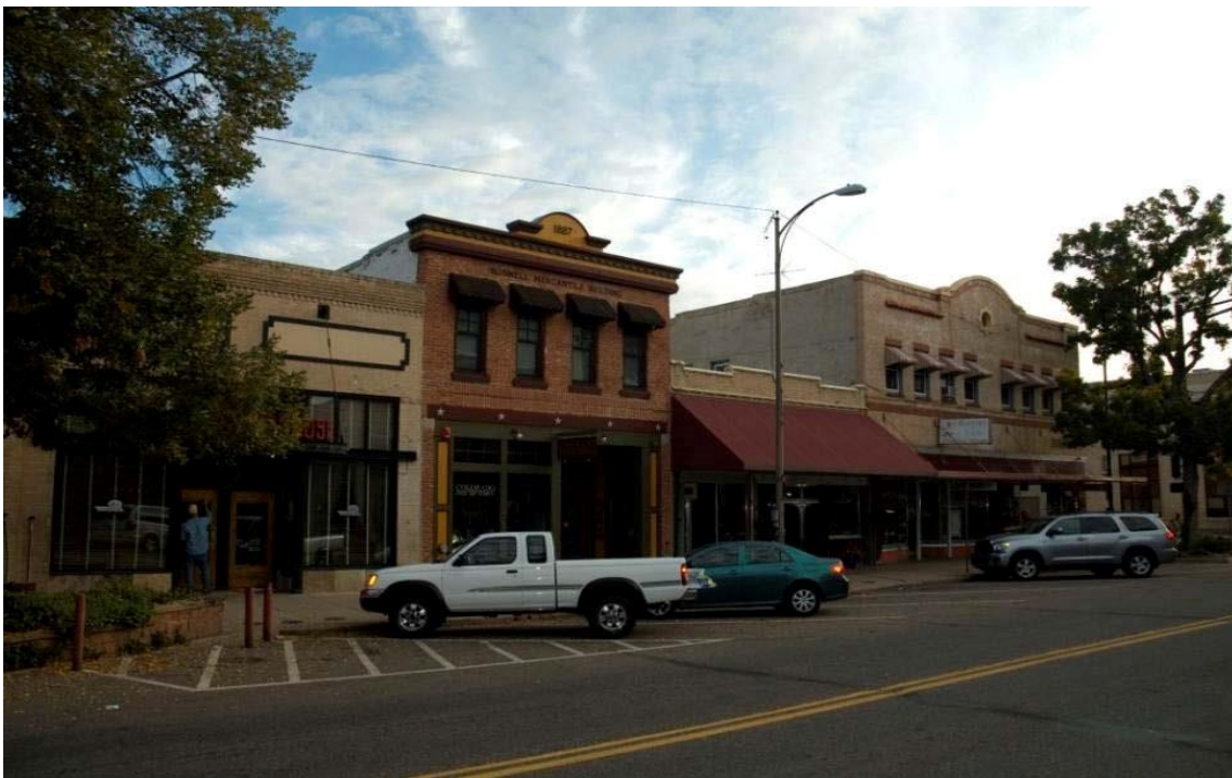
Photo 12: Camera facing northeast - 125 East 4th Street, 129 East 4th Street, 133/135 East 4th Street, 137/141 East 4th Street - 5LR.5077 C, 5LR.6175 NC, 5LR.5075 C, 5LR.1054 C
