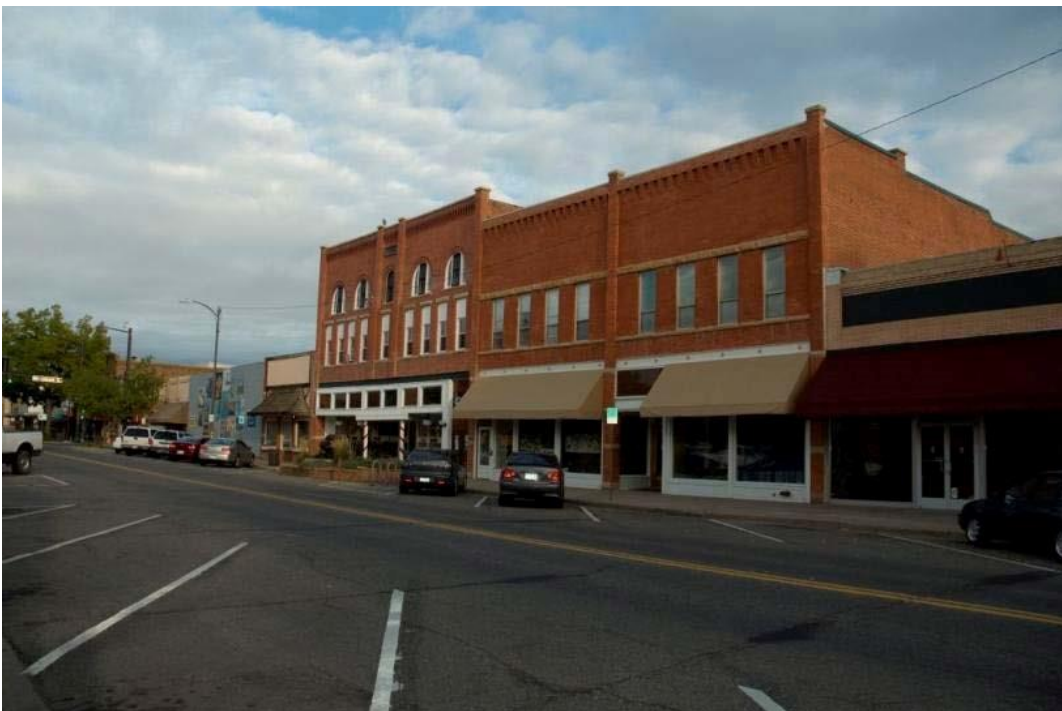
Photo 2: Camera facing northwest - 315/319 East 4th Street, 325/333 East 4th Street, 337 East 4th Street – 5LR.5091 C, 5LR.5090 C , 5LR.5089 C
