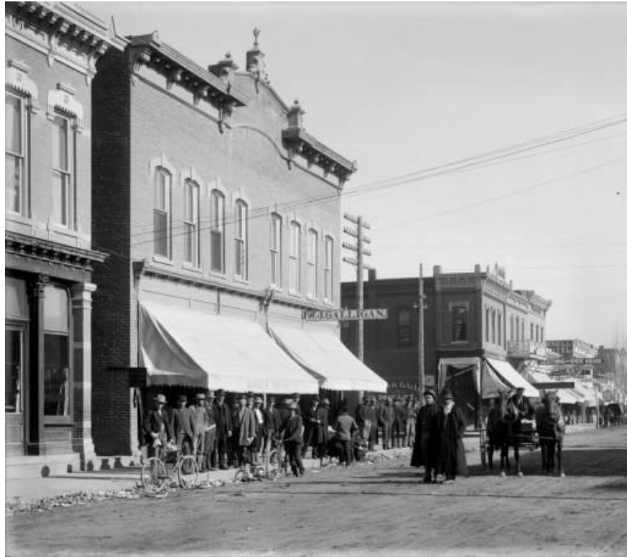
Figure 4: E. 4 th St. at N. Cleveland Ave., view to NE, ca. 1905. Courtesy Loveland Public Library, Loveland, Colorado.
