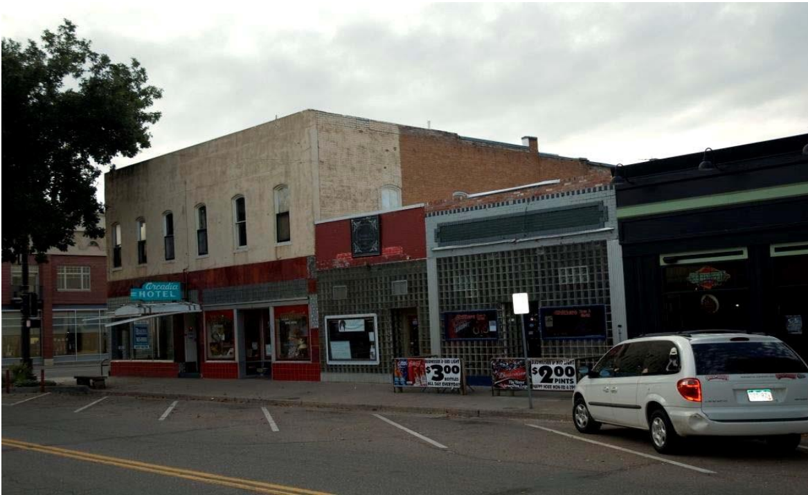
Photo 17: Camera facing southeast - 128 East 4th Street, 134 East 4th Street, 136/138/140 East 4th Street - 5LR.6182 C, 5LR.6183 C, 5LR.1056 C
