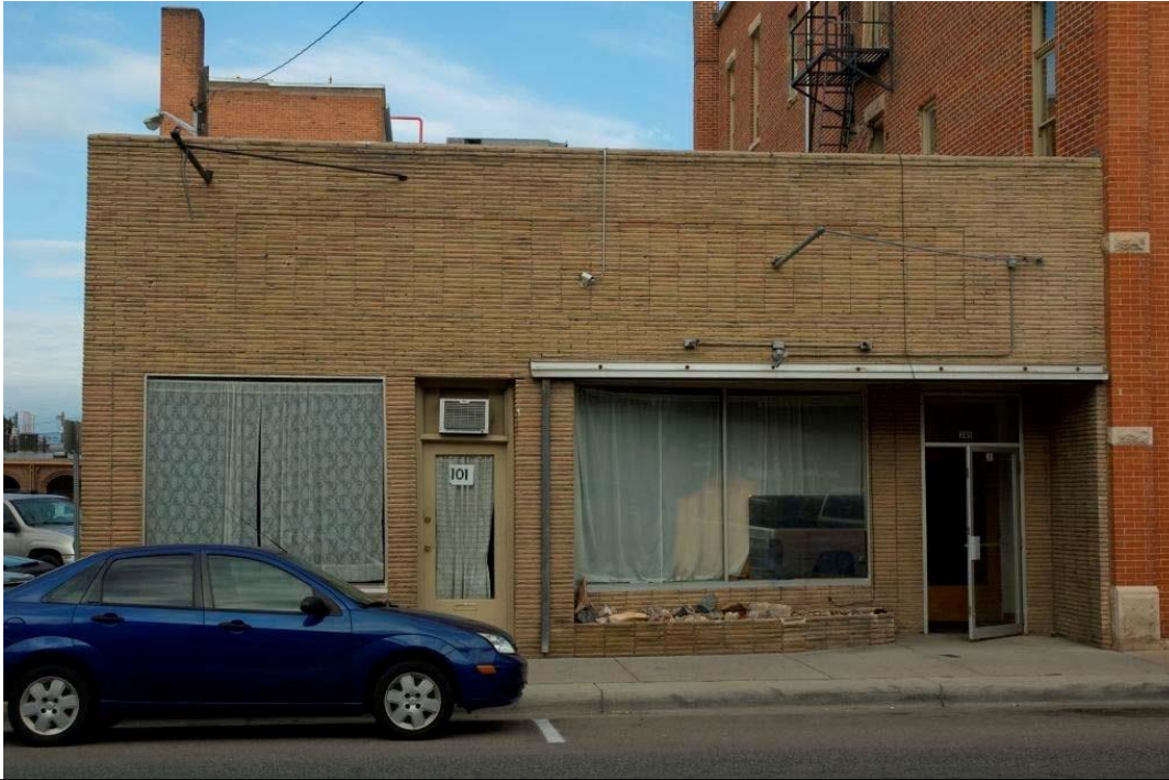
Photo 25: Camera facing west - 365 N. Lincoln Avenue – 5LR.9612 C
