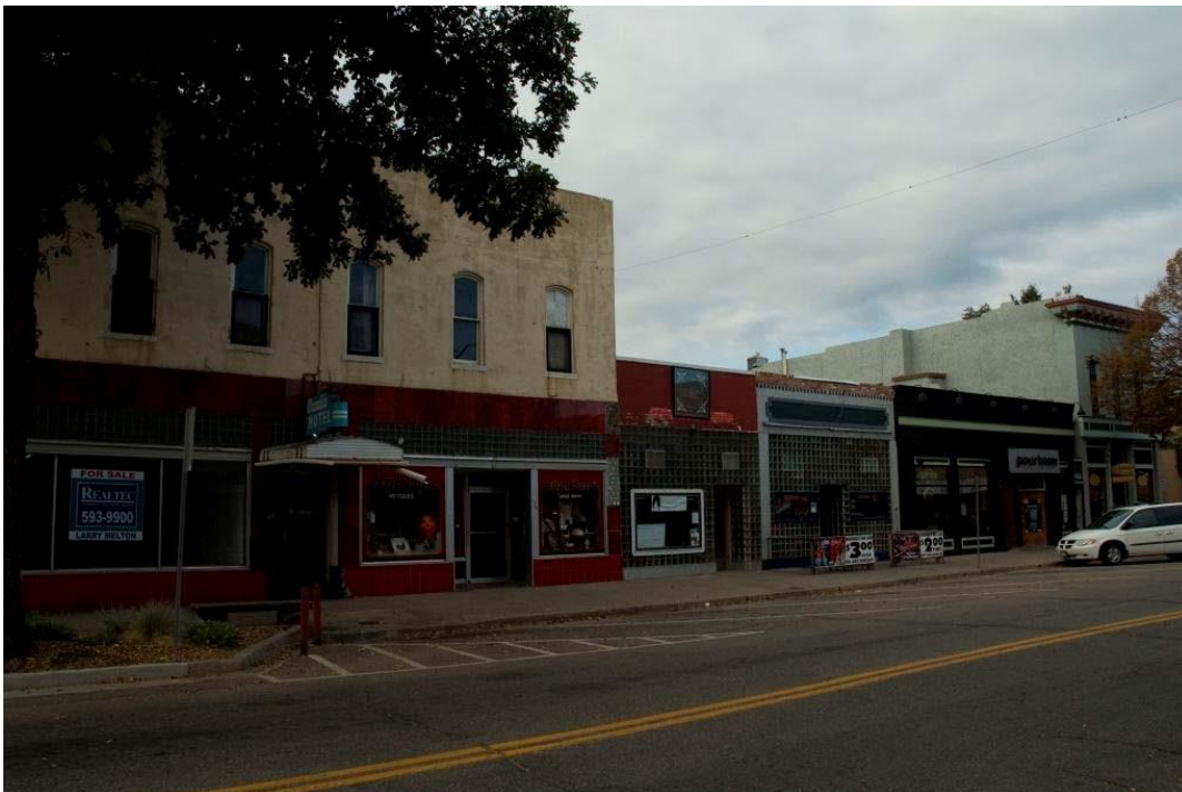
Photo 28: Camera facing southwest - 120/122 East 4th Street, 124 East 4th Street, 128 East 4th Street, 134 East 4th Street, 136/138/140 East 4th Street – 5LR.5065 C , 5LR.6181 NC, 5LR.6182 C, 5LR.6183 C, 5LR.1056 C
