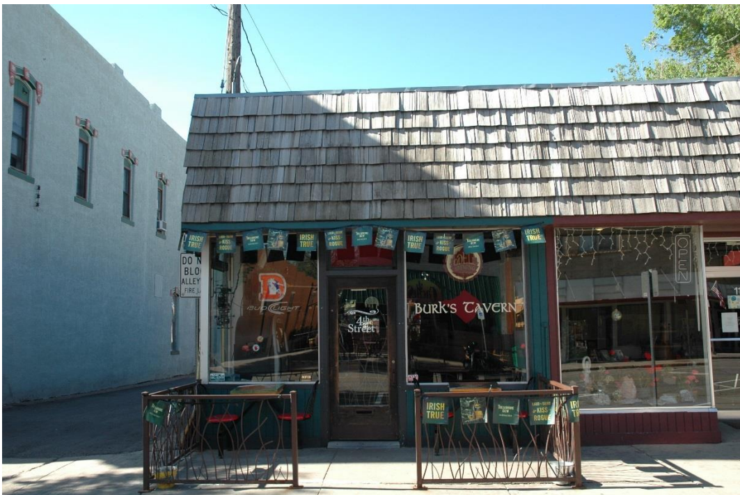
Photo 36: Camera facing south – 116/118 East 4 th Street, 5LR.6179 C
