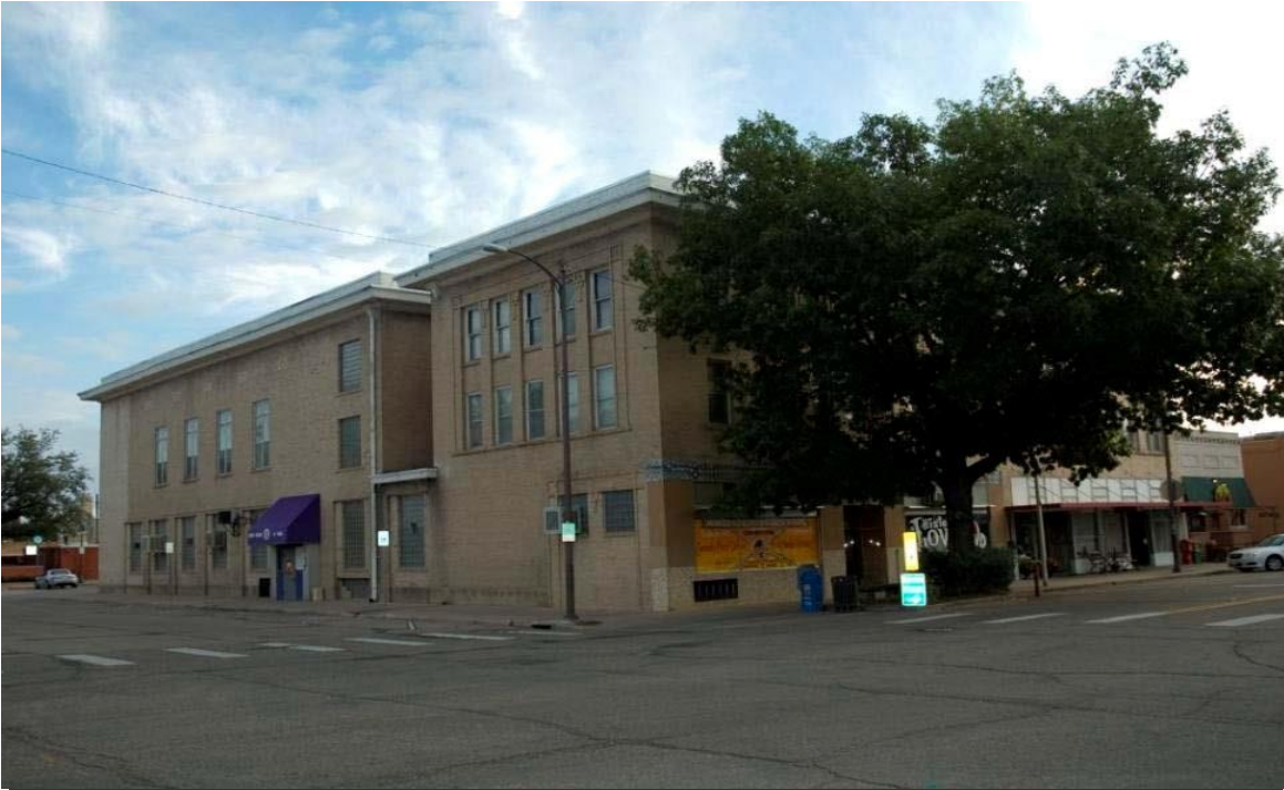
Photo 13: Camera facing northeast - 103/111/117 East 4th Street - 5LR.685 C
