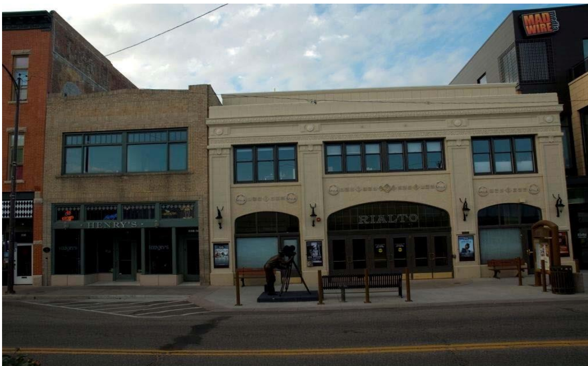
Photo 20: Camera facing south - 228 East 4th Street, 234 East 4th Street - 5LR.1058 C, 5LR.5069 C
