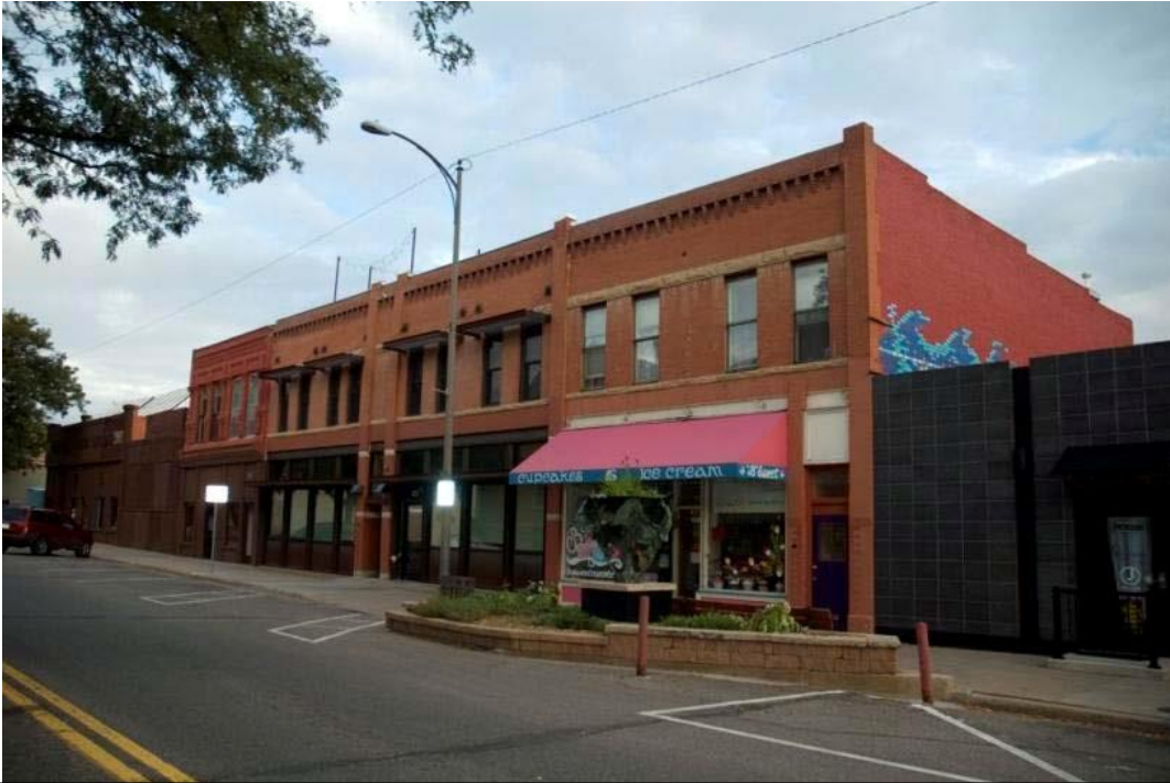
Photo 1: Camera facing northwest - 403 East 4th Street ---- East 4th Street, 415 East 4th Street, 419/425 East 4th Street - 5LR.5086 NC, 5LR.13320 NC, 5LR.13321 NC, 5LR.9749 C
