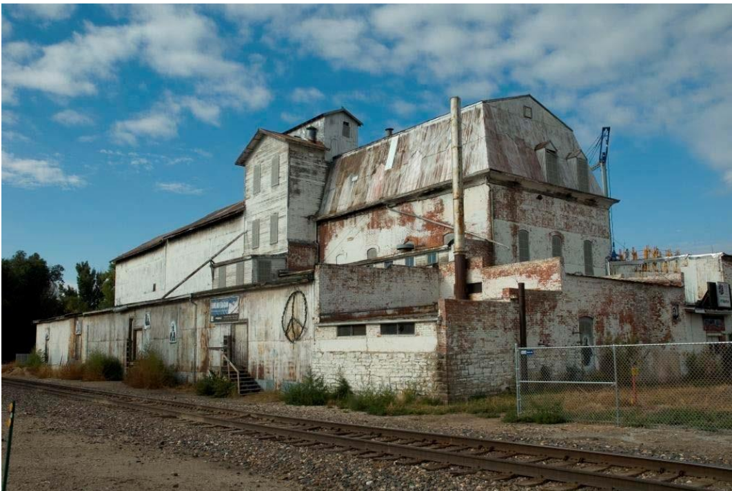
Photo 32: Camera facing southwest - 130 W. 3rd Street – 5LR.6671 C
