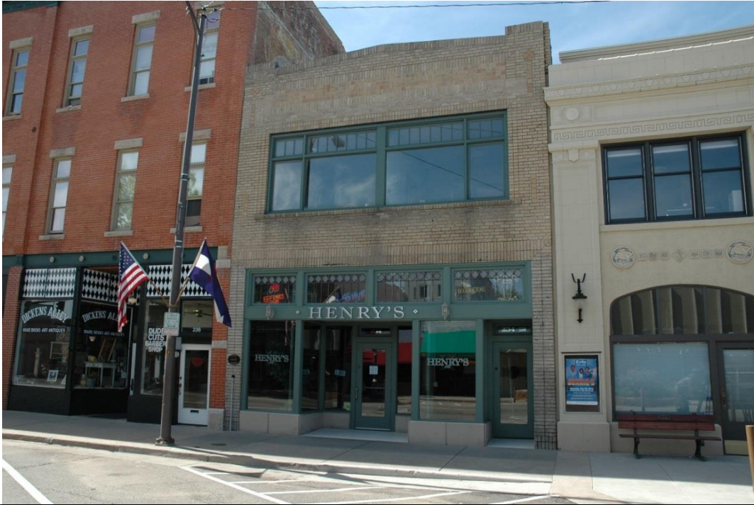
Photo 39: Camera facing south-southeast – 234 East 4 th Street, 5LR.5069 C
