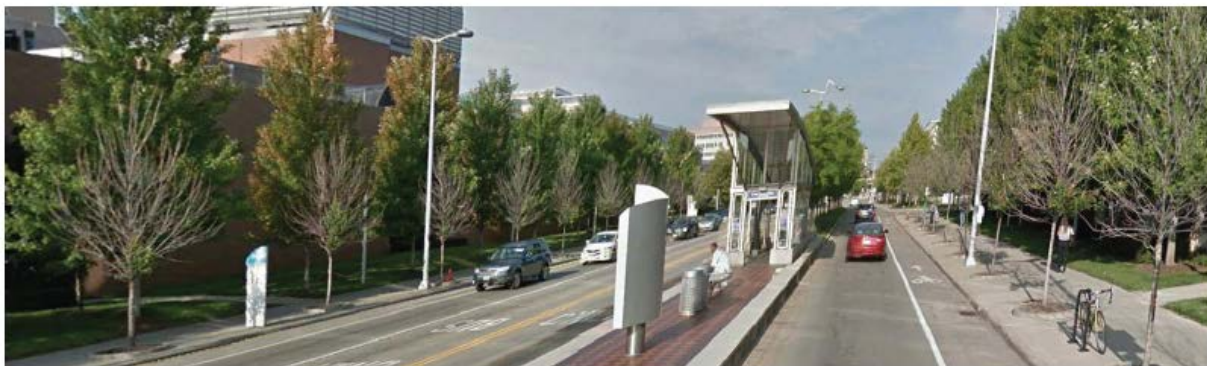
Sidewalk | 2 Bus Lanes with 1 Vehicle Lane | Median | Vehicle Lane | Bike Lane | Sidewalk | Right of Way 100'
