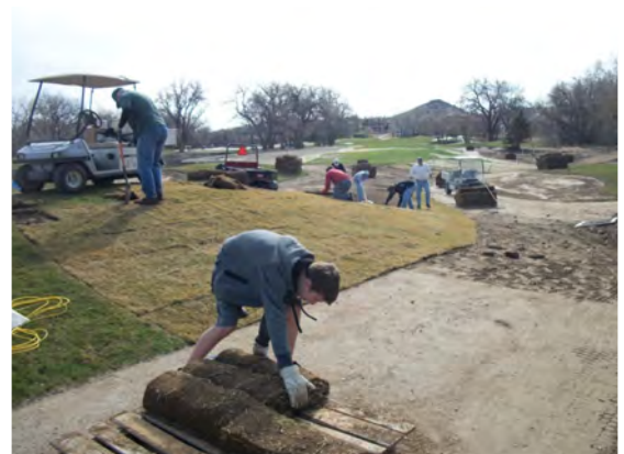
Mariana Butte Flood Repairs
