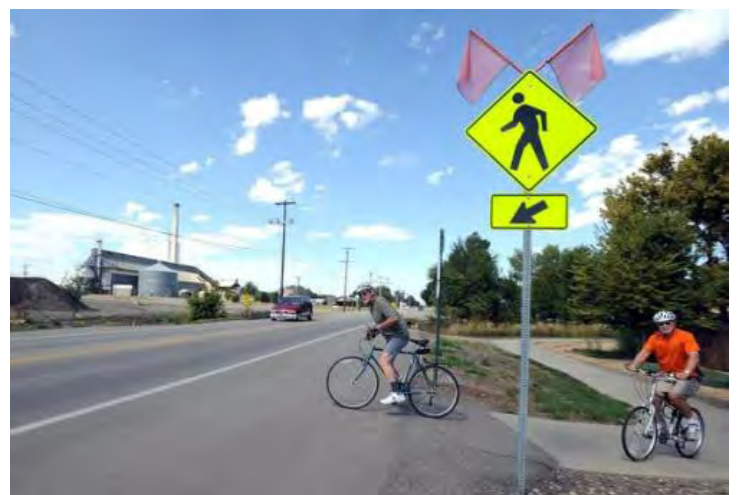
Madison Avenue Trail (location of under-construction pedestrian trail underpass)
