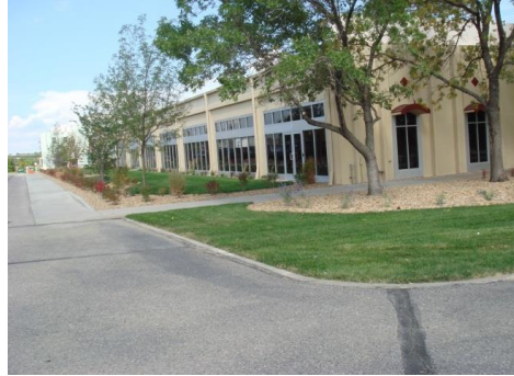
619 14th Street SW following renovation
