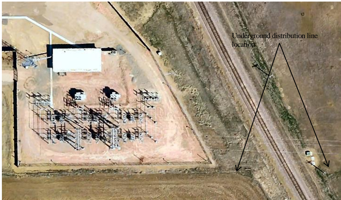
Figure 2: Horseshoe Substation and distribution line.
