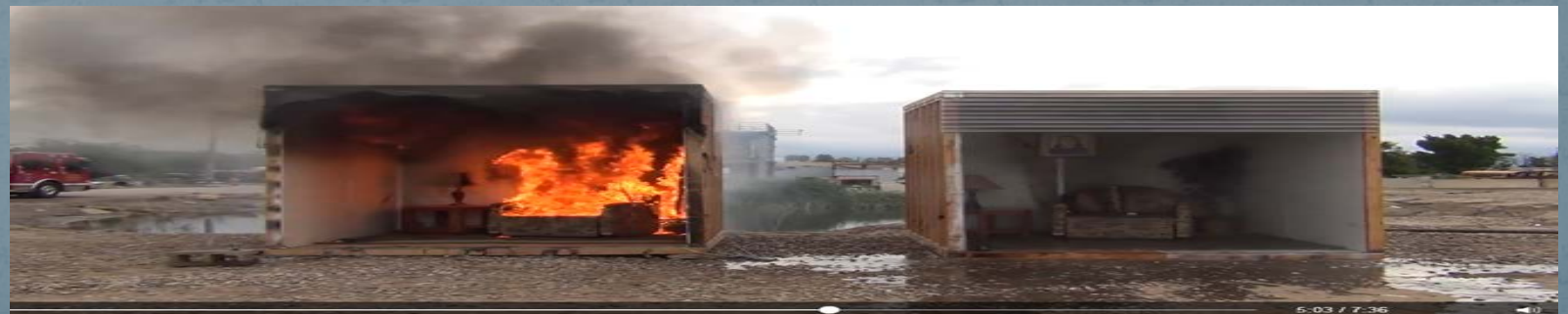
Fire in left burn cell at 5:03 – complete loss of all furnishings in the left cell and fire continuing to progress
