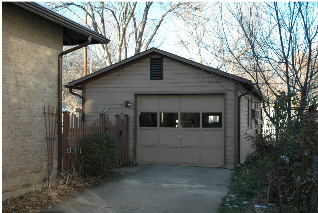
Figure 3: Garage South (Front) Elevation
