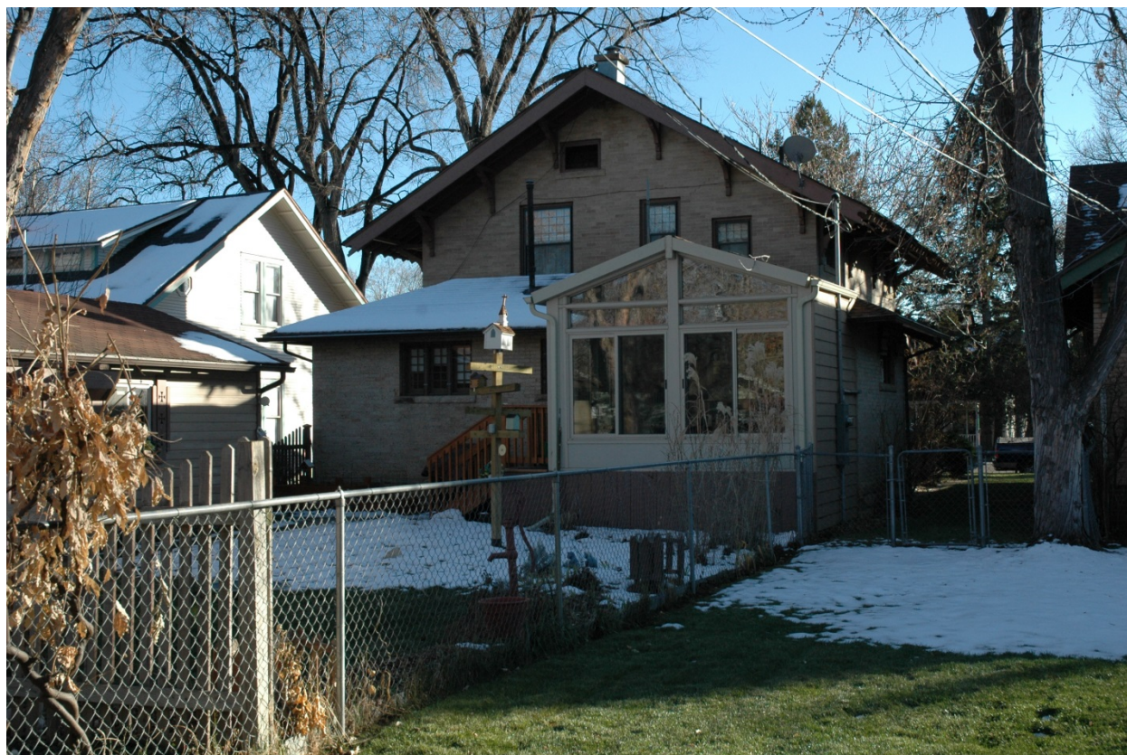
Figure 4: North (Rear) Elevation
