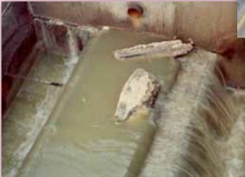
Above: Chunks of grease that arrived at the wastewater treatment plant. Bottom right: Pipe clogged with grease.
