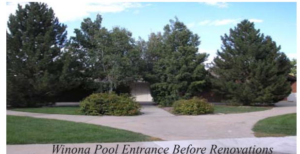
Winona Pool Entrance Before Renovations
