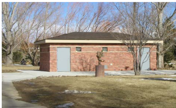
New Restroom Building at Benson Sculpture Garden
