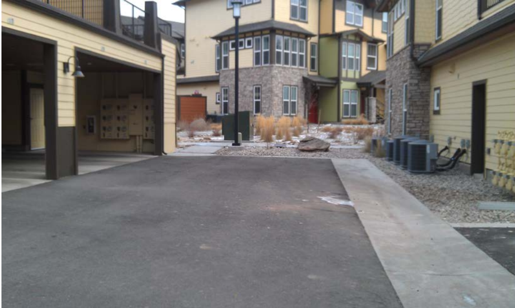
Looking northeast along drive aisle; esmt overlap area is on left side; currently there are no "No Parking Fire Lane" signs on the right (easterly) side
