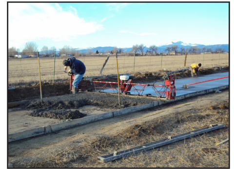
Concrete work on Recreation Trail
