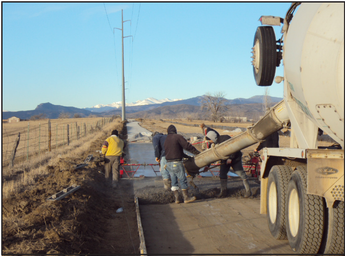
Crews pouring concrete on Recreation Trail Segment 6b
