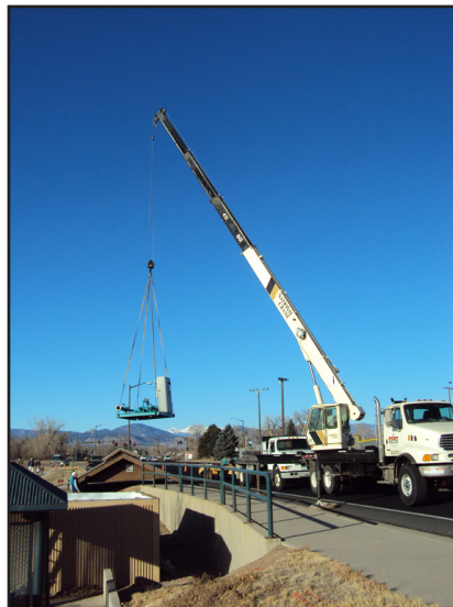
Replacement of Irrigation Pump at Centennial Park
