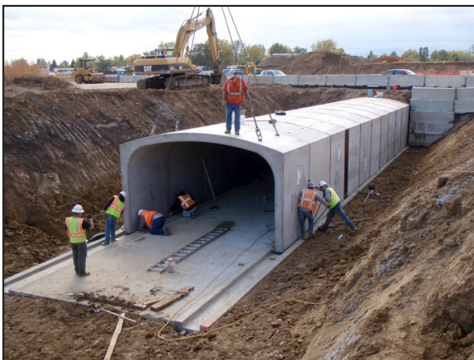
Placement of boxes for Highway 287 Recreation Trail Underpass
