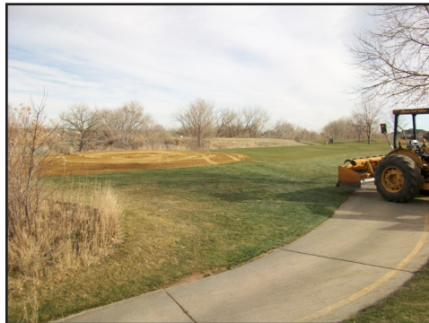
Mariana Butte Golf Course Construction of Championship Tee Box
