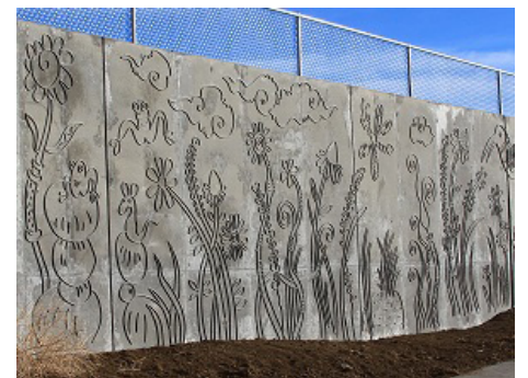
Concrete Art Installed at Highway 287 Underpass
