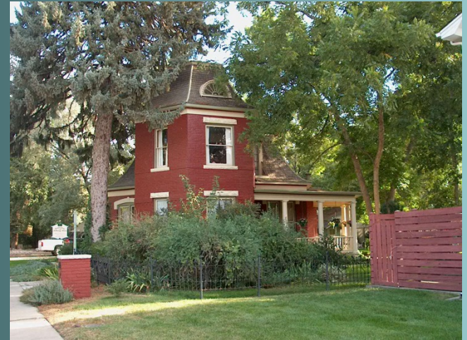
McCreery House, 746 N Washington Ave
