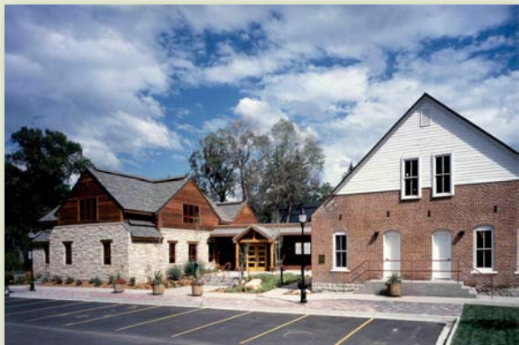
Centennial Hall-Carver Power Plant in Steamboat Springs (photo courtesy of John Robledo)
