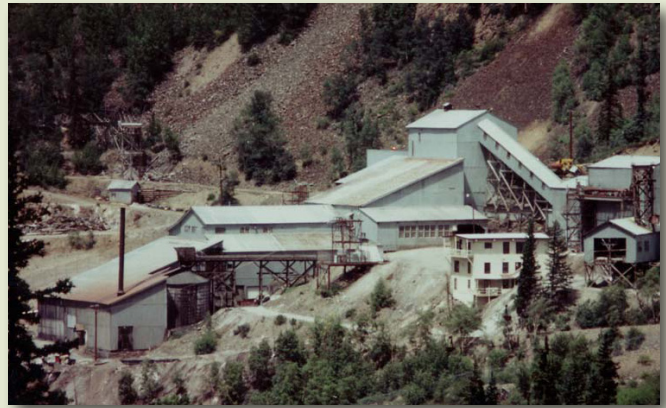
Historic Shenandoah-Dives Mill
