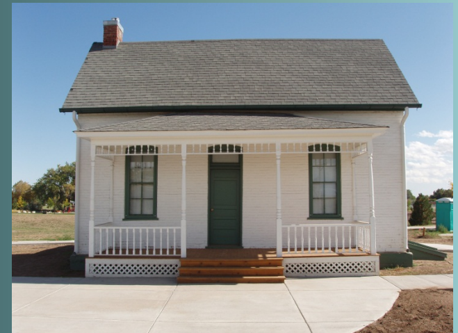
710 S Railroad Avenue
