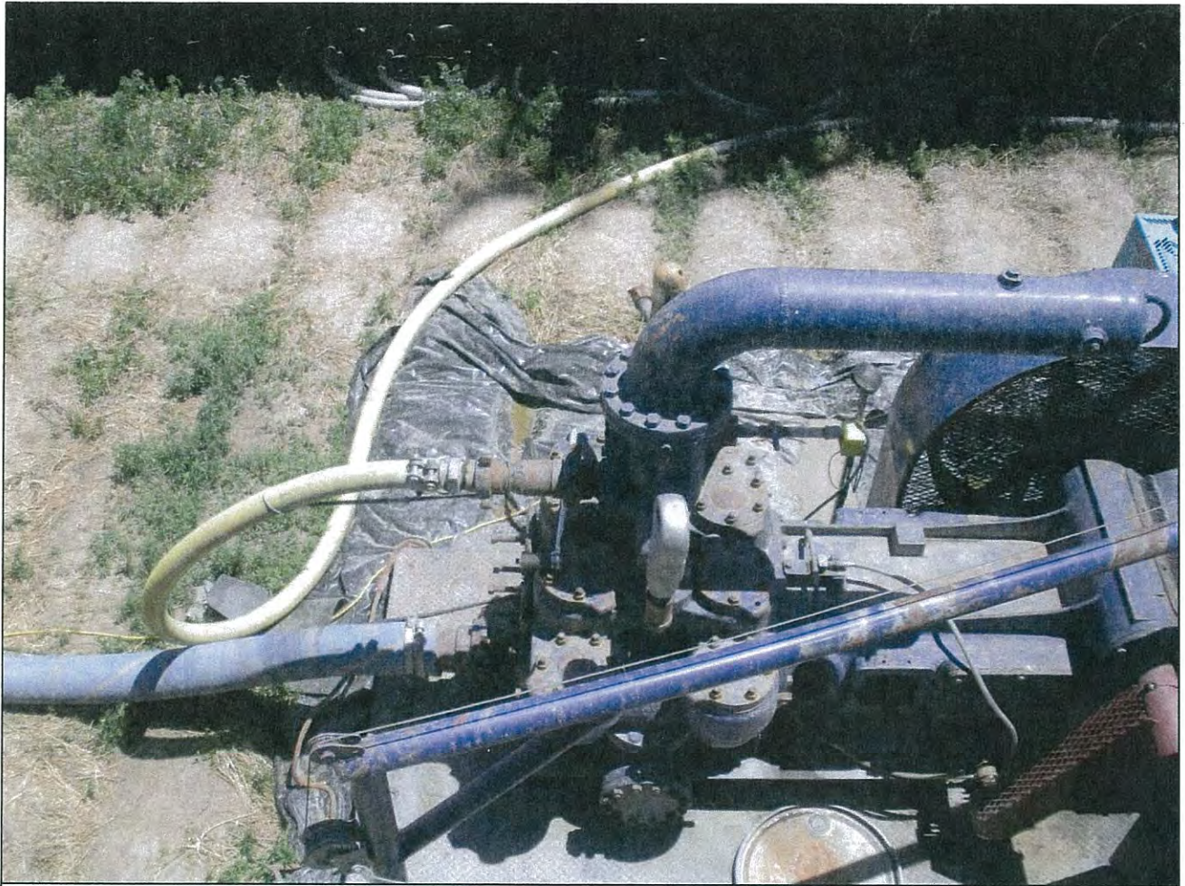
Figure C15. Photograph of pumping of mud back to borehole at MW02.
