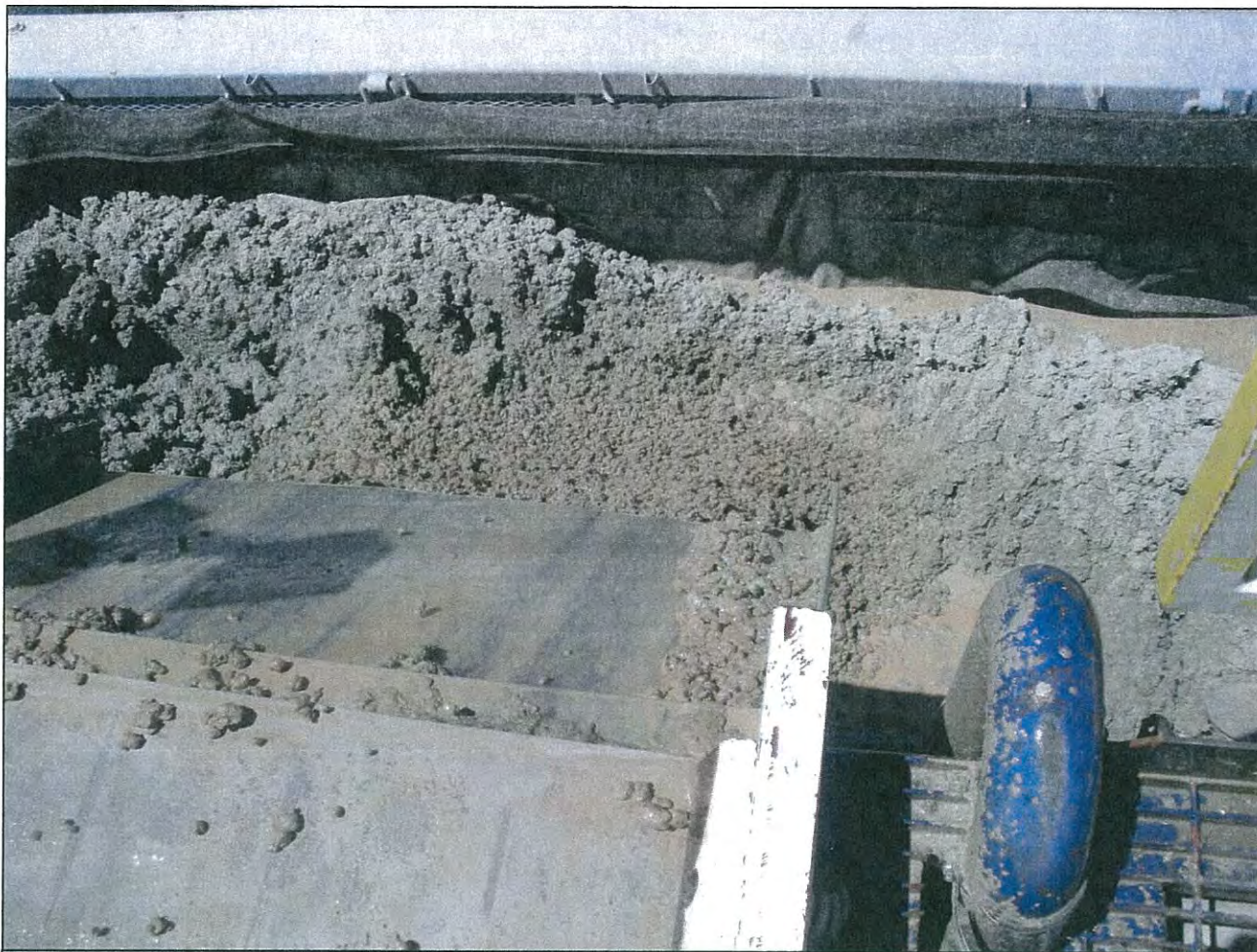
Figure C14. Photograph of cuttings transported to disposal bins at MW02.
