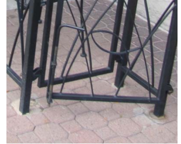
Figure 6. Railing installed in sleeves
