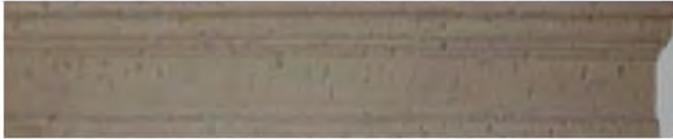
PRECAST CORNICE SILLS AND WALL BASE
