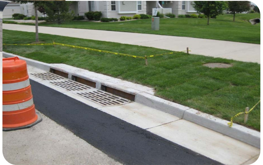
Inlet/manhole connection after installation.
