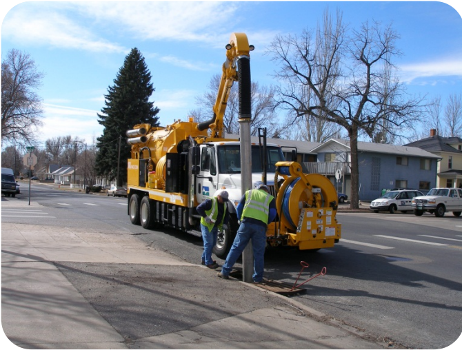
VacCon crew jetting storm drains.
