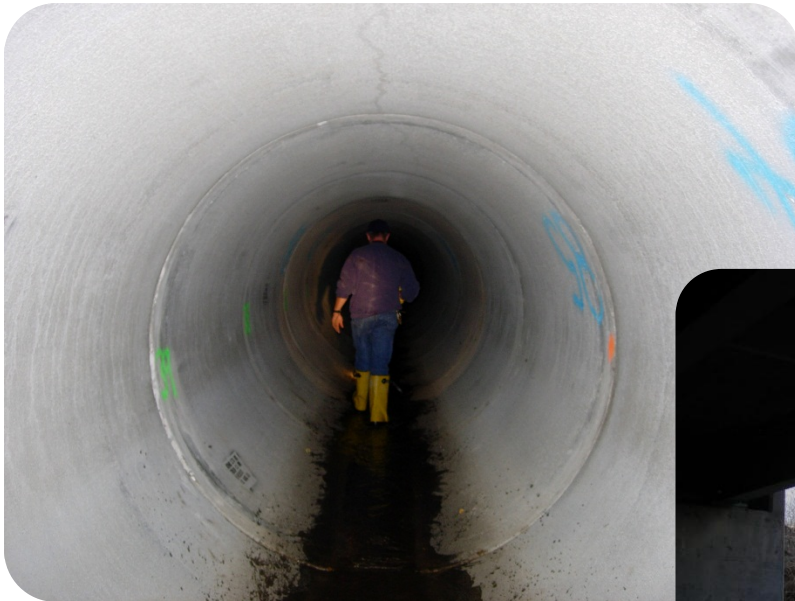
Above, crews inspect a 6 foot storm sewer. At right, crews remove a blockage at the Big Thompson River.
