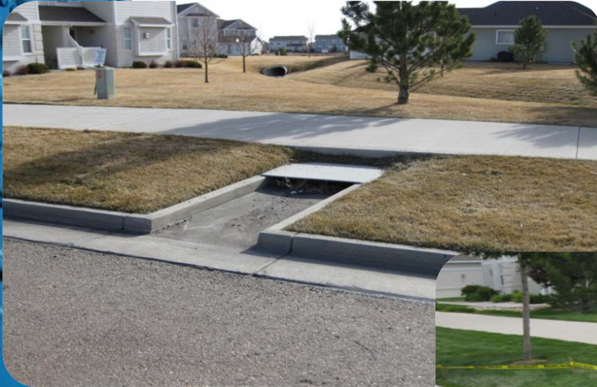
Curb cut/manhole connection before installation
