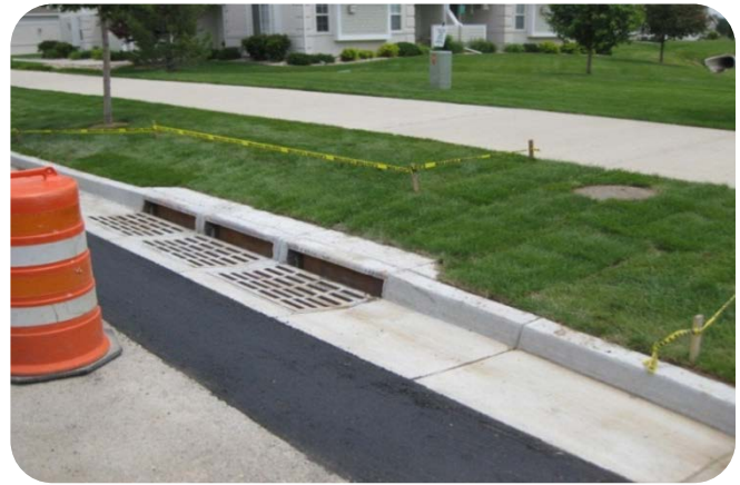
Inlet/manhole connection after installation.
