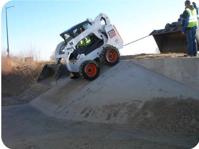
Crews use a bobcat to clean a ditch vault
