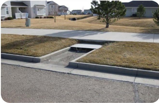
Curb cut/manhole connection before installation
